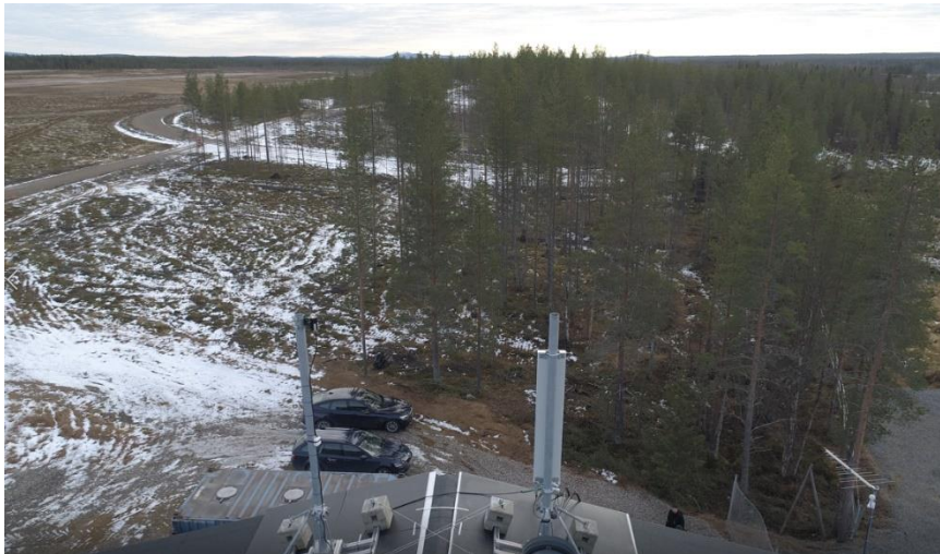
Figure 4. 5G test network base station antenna and the test track.
